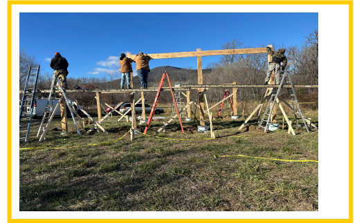
Construction begins on RVF's new learning pavilion
